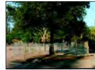
IMAGE 2.15-2 Tree Protection Fence at the Dripline
