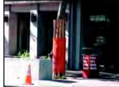
IMAGE 2.15-4 Trunk Wrap Protection
