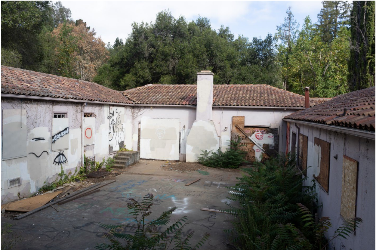
Figure 1 - View of courtyard, looking northwest.
