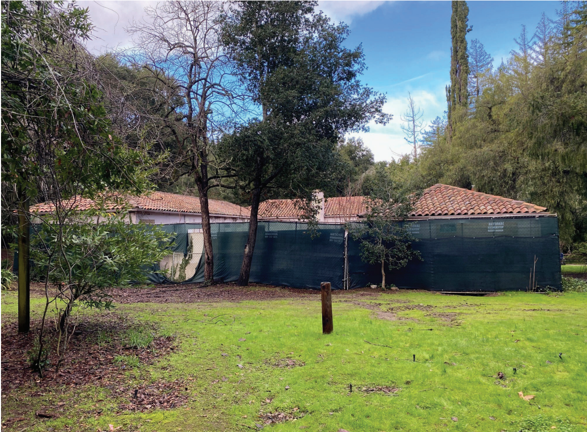
Photo 1: Photo of existing building.
