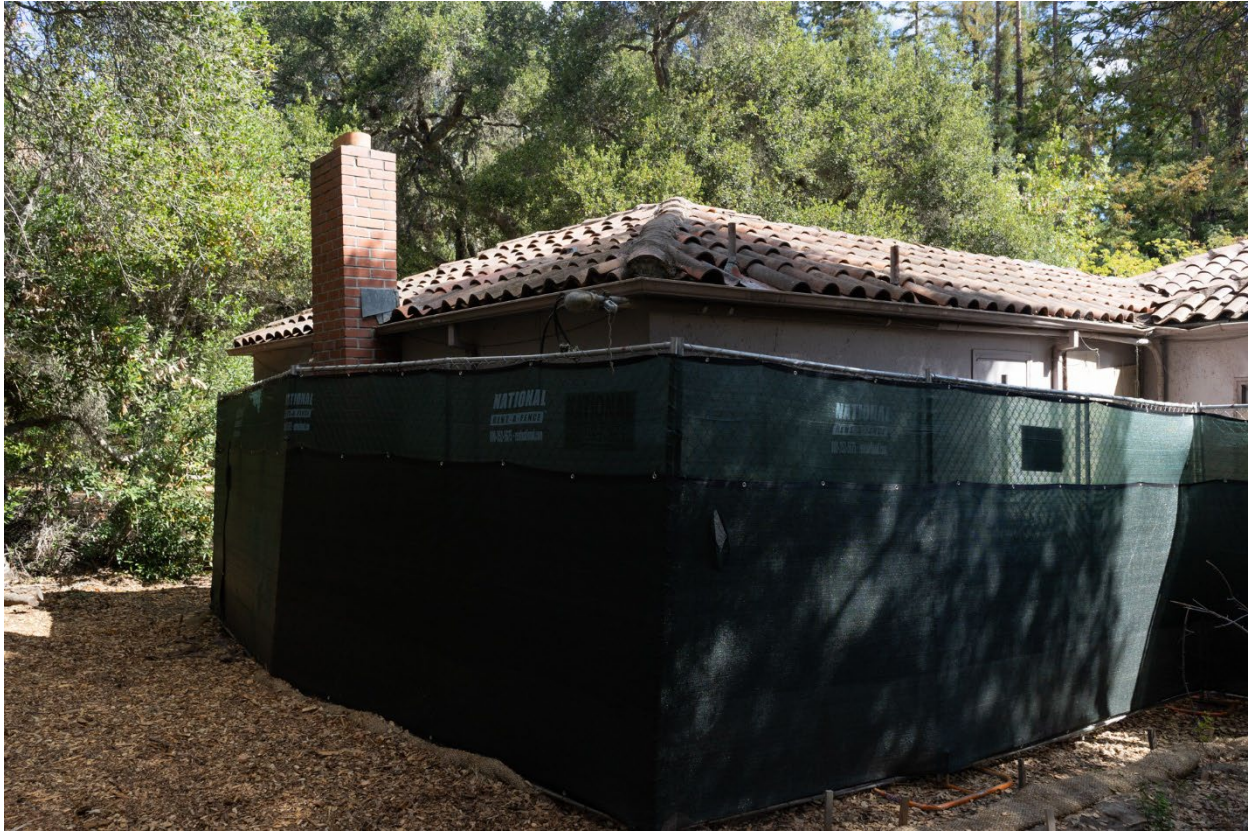
Figure 2 - View of the brick chimney at west addition, view looking northeast.
