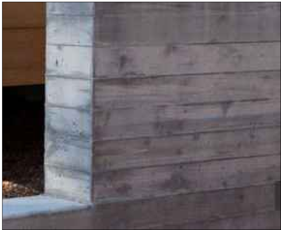
BOARD FORMED CONCRETE
