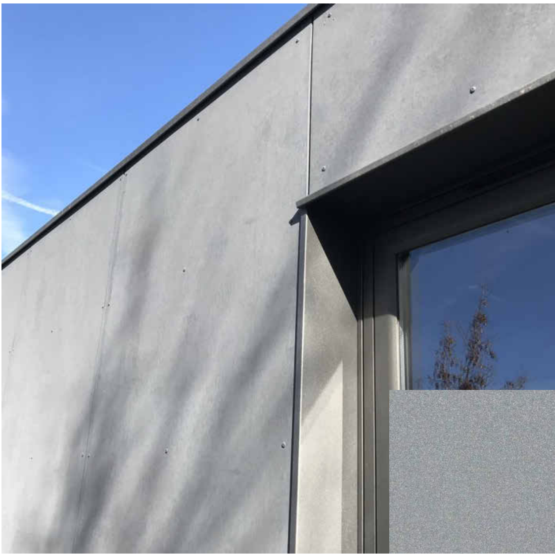
MT 2 - METAL WALL PANEL WESTERN STATES METAL ROOFING - T-GROOVE - ZINC METALLIC
