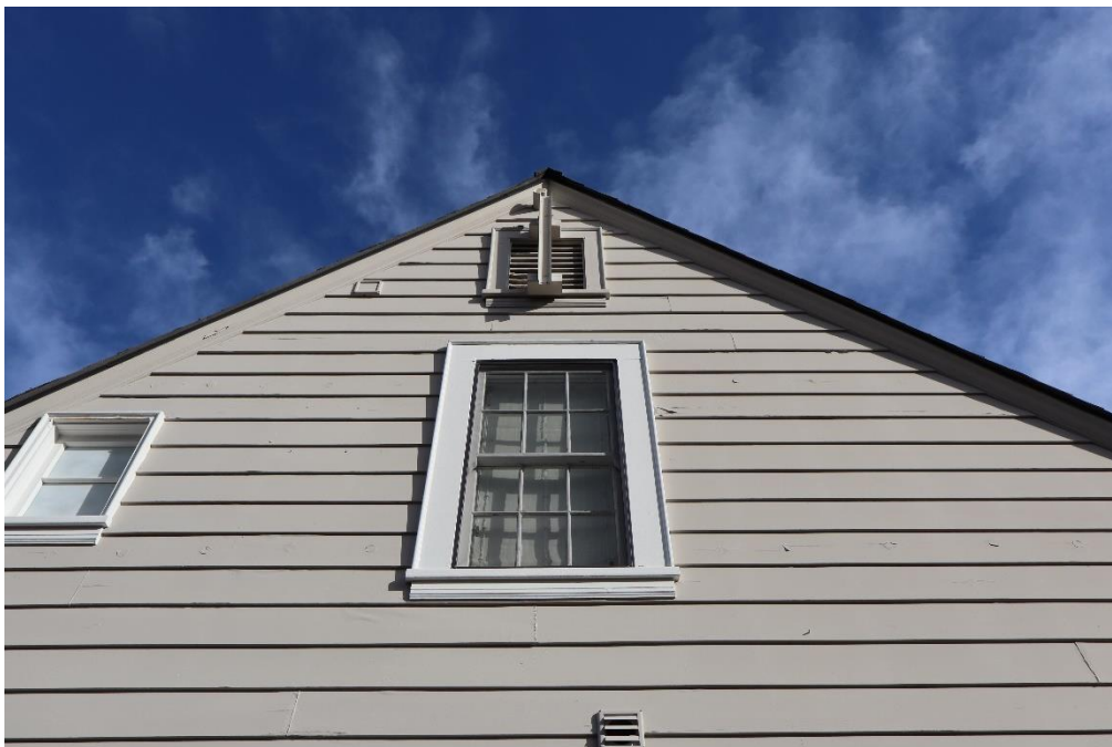
Figure 22. West elevation gable.
