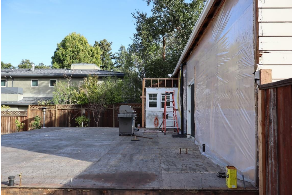
Figure 23. North elevation, facing east.
