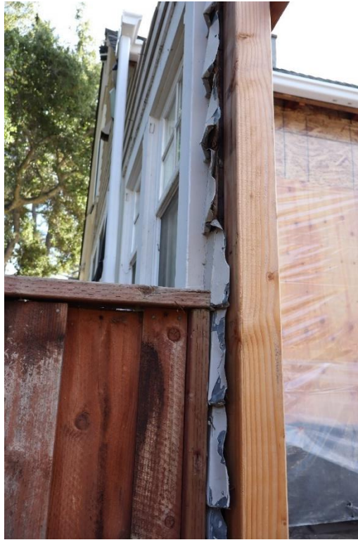
Figure 25. Photograph showing a portion of an addition, no longer extant.
