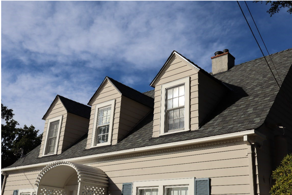
Figure 4. Photograph showing the three roof dormers.
