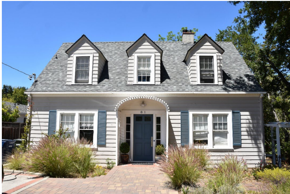
Figure 15. Primary (south) façade, view north.
