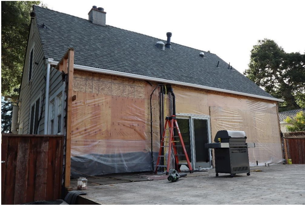
Figure 24. North elevation, facing south.
