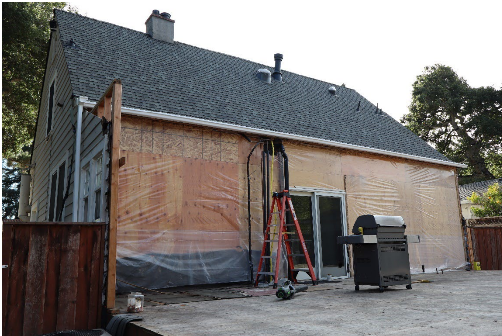
Figure 8. North elevation, facing south.
