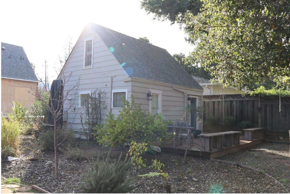
Figure 13. Photograph showing the north and east elevations, facing southwest.
