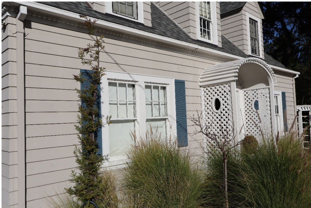
Figure 3. Photograph showing a pair of windows along the primary façade.
