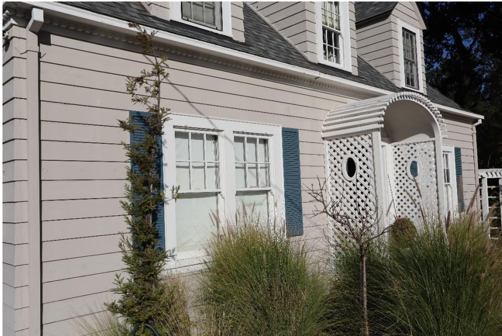
Figure 19. Photograph showing a pair of windows along the primary façade.
