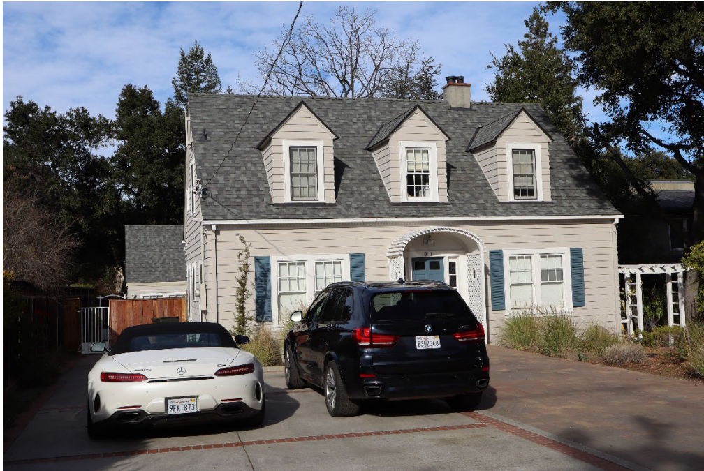
Figure 2. Primary façade, facing north.
