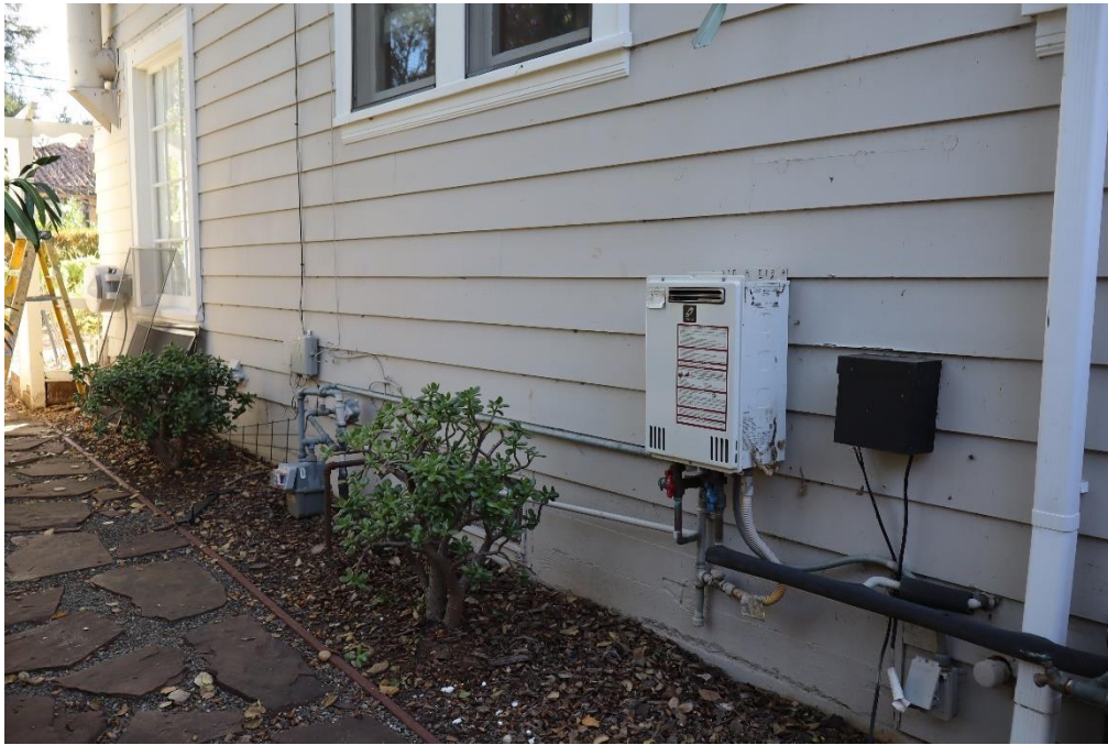
Figure 27. Photograph showing the board-formed concrete foundation is exposed along this elevation.
