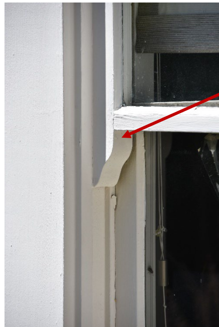
Figure 18. Detail of ogee lug on double-hung wood window.
