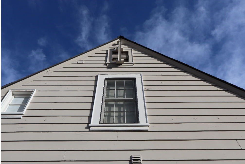
Figure 6. West elevation gable.
