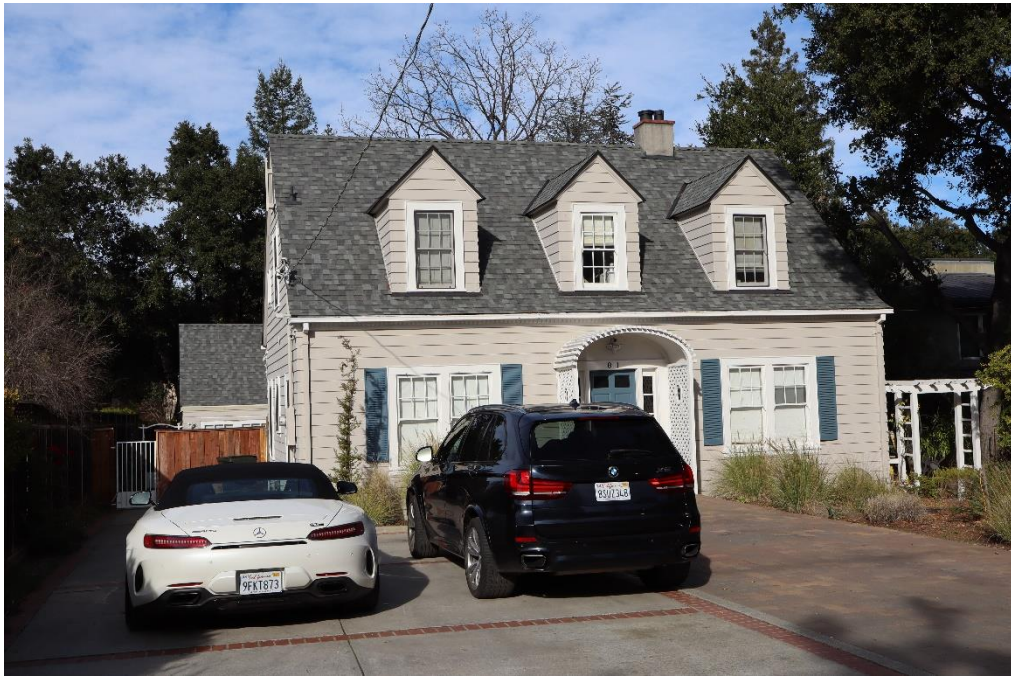
Figure 18. Primary façade, facing north.
