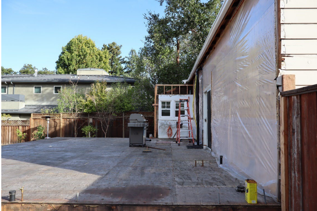
Figure 7. North elevation, facing east.
