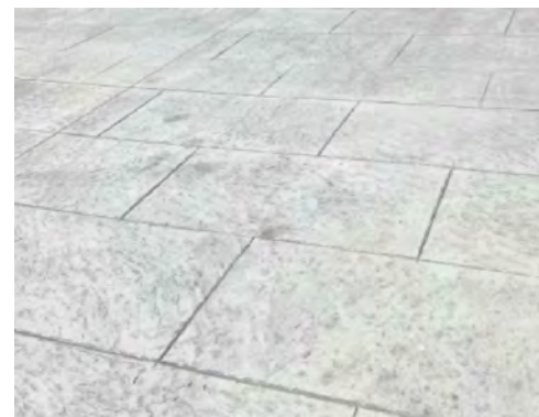
CONCRETE VEHICULAR SIDEWALK STAMPED, NAT. GRAY
