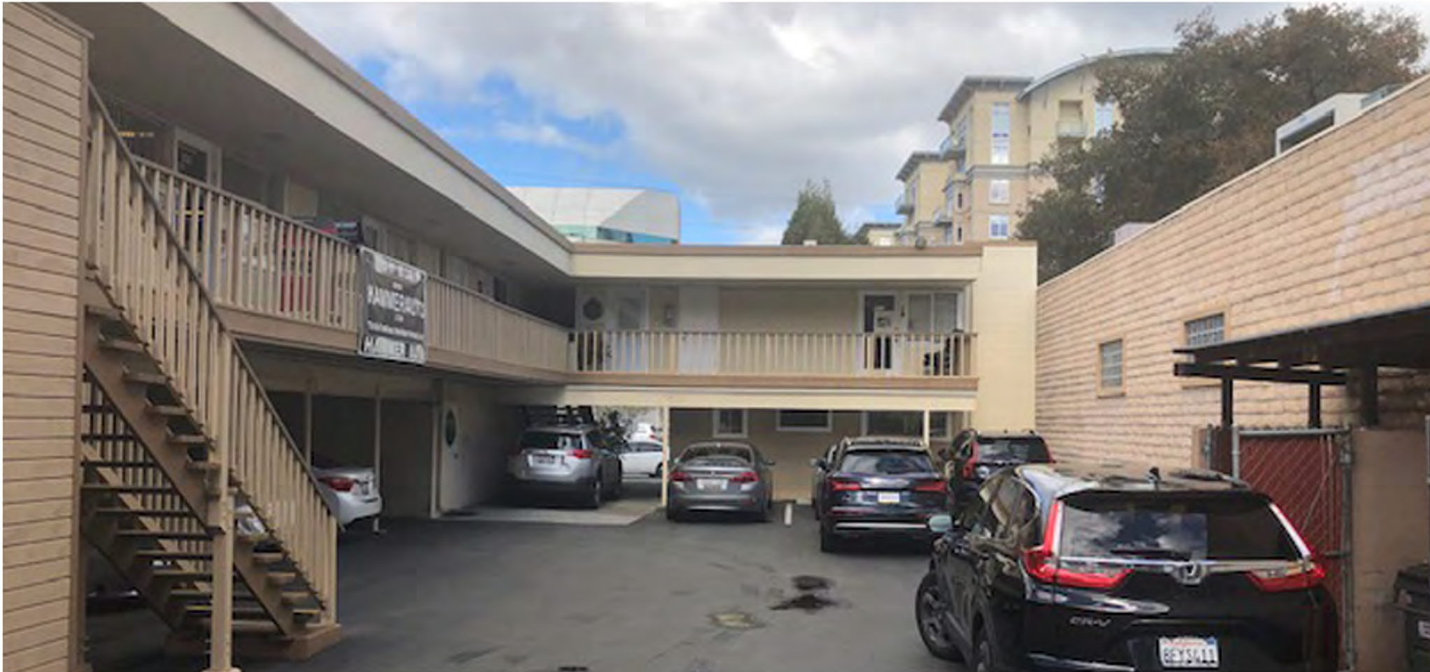
VIEW OF EAST SIDE OF BUILDING
