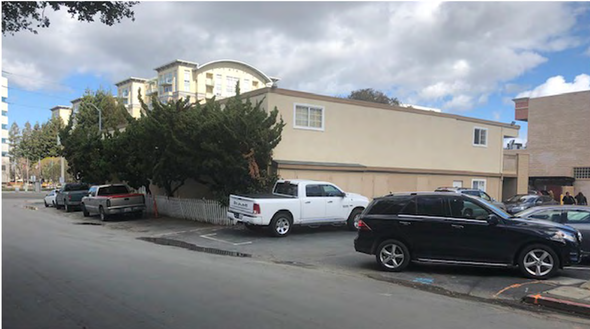
VIEW FROM JORDAN AVE. - REAR
