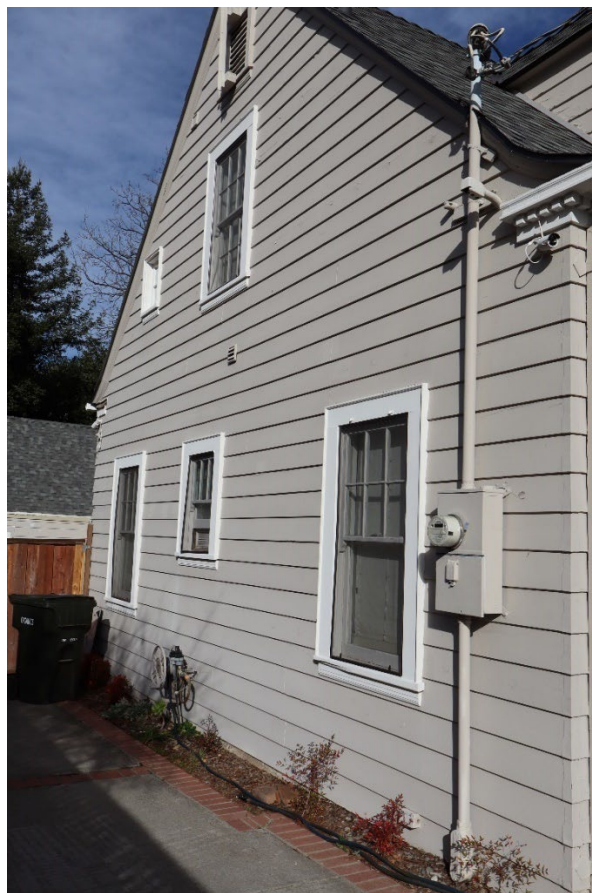
Figure 5. West elevation, facing north.
