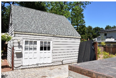
Figure 7. Garage/Cottage at northwest corner of property, south façade.
