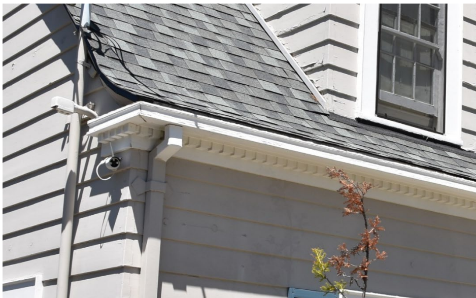
Figure 16. Primary façade, detail of cornice with dentils and eave return.
