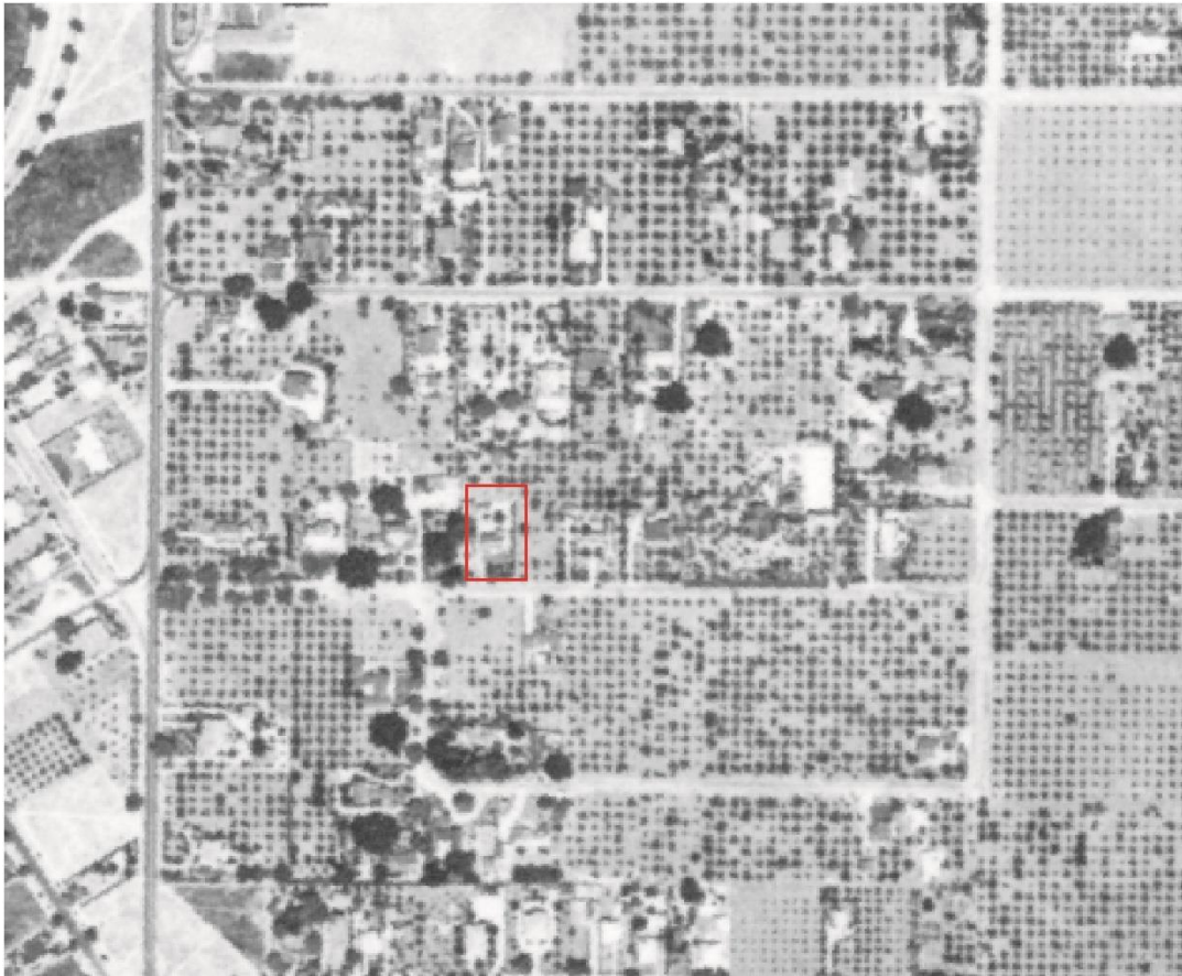
Figure 16. 1939 aerial, showing the 1929 house and ca. 1933 detached garage within the Property (courtesy of University of Santa Barbara Library).
