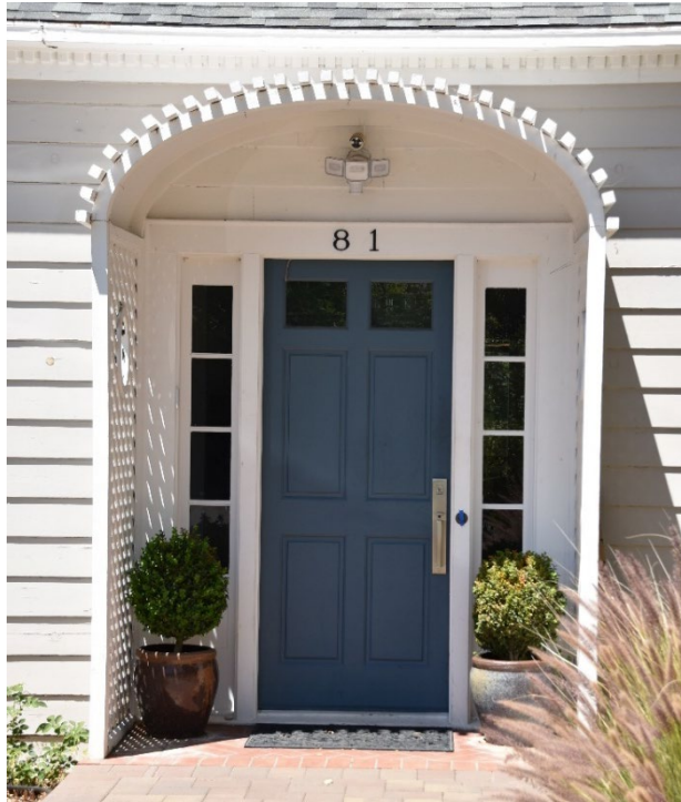
Figure 17. Detail of front entry.
