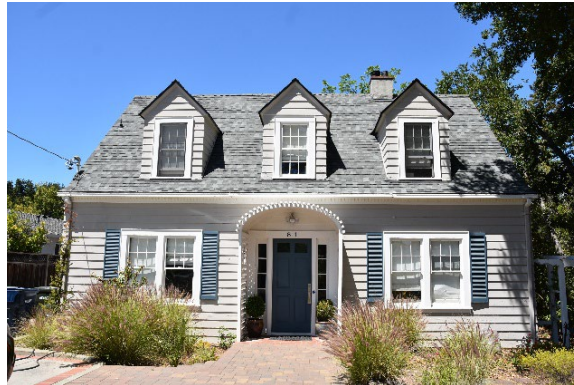
Figure 4. South (front) façade, view north.
