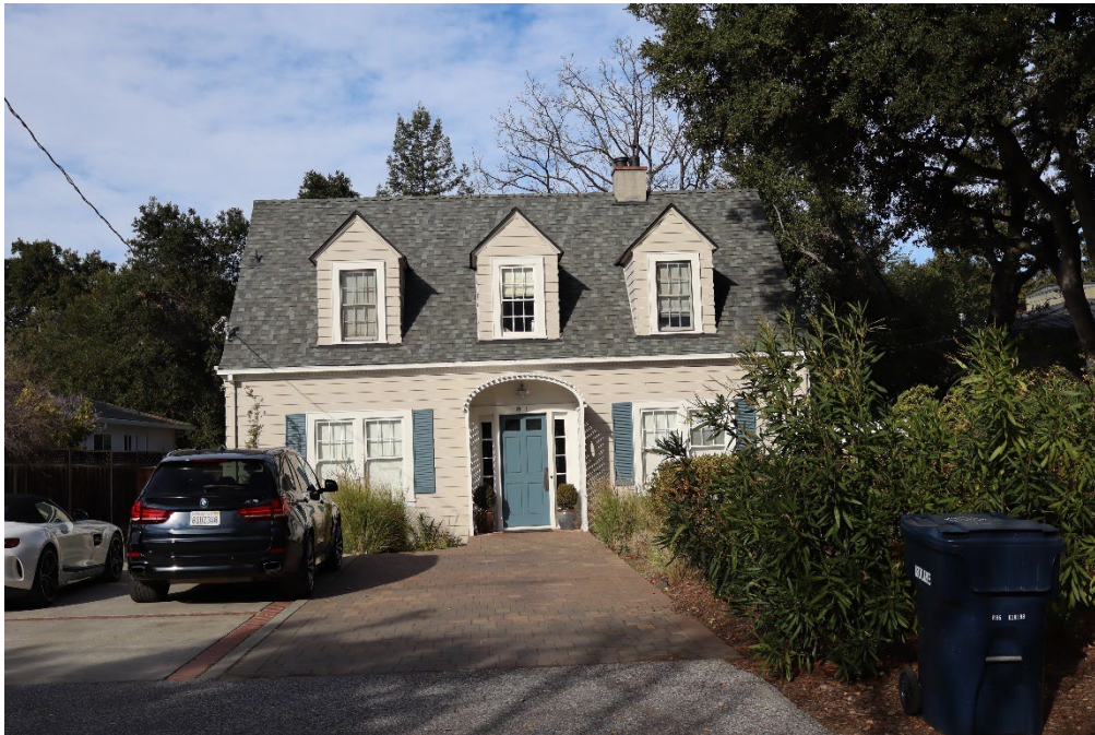
Figure 1. South elevation, facing north.
