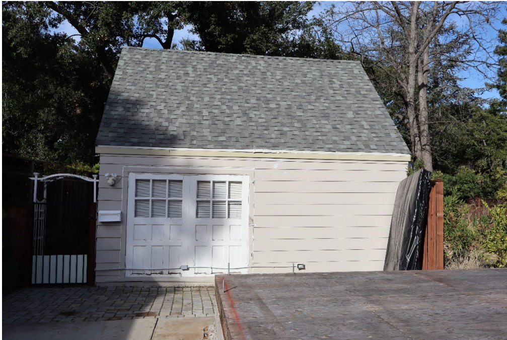
Figure 12. South elevation, facing north.
