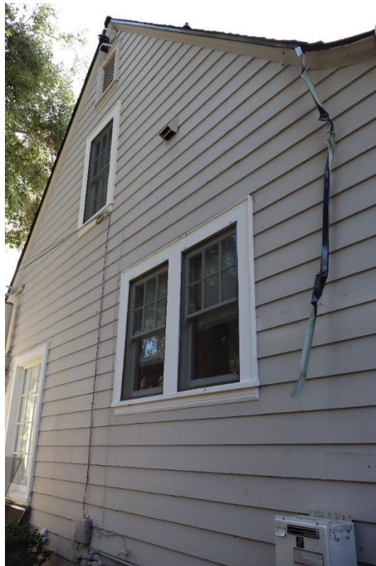
Figure 26. The east façade, facing south.
