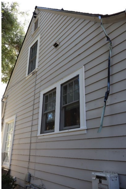
Figure 10. The east façade, facing south.
