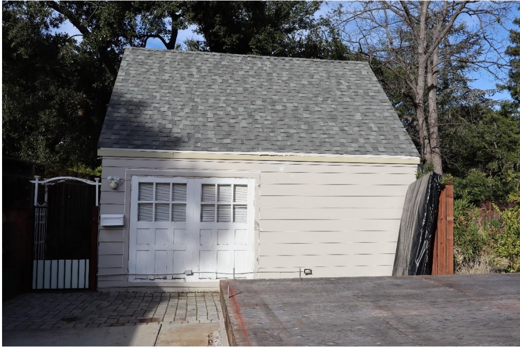
Figure 28. South elevation, facing north.
