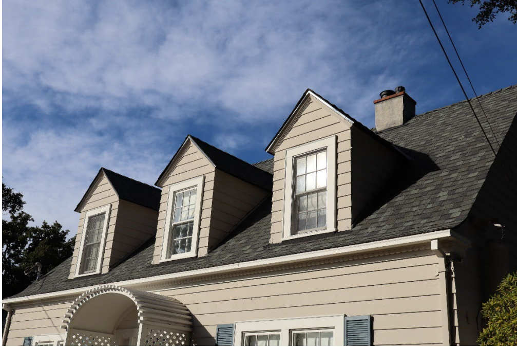
Figure 4. Photograph showing the three roof dormers.
