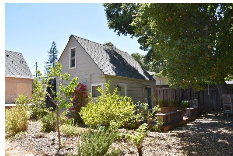
Figure 8. Garage/Cottage at northwest corner of property, east and north facades.
