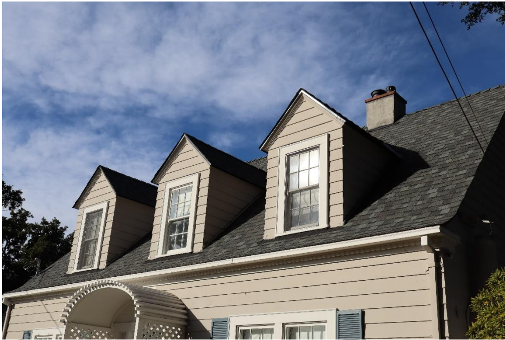
Figure 20. Photograph showing the three roof dormers.
