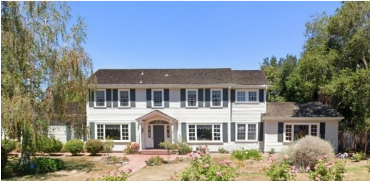
Figure 14. 1570 Kensington Circle Source: Google Streetview.
