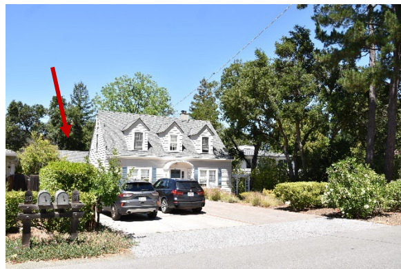
Figure 6. Long view of south façade of property from Pepper Drive. Roof of garage/cottage indicated by red arrow.
