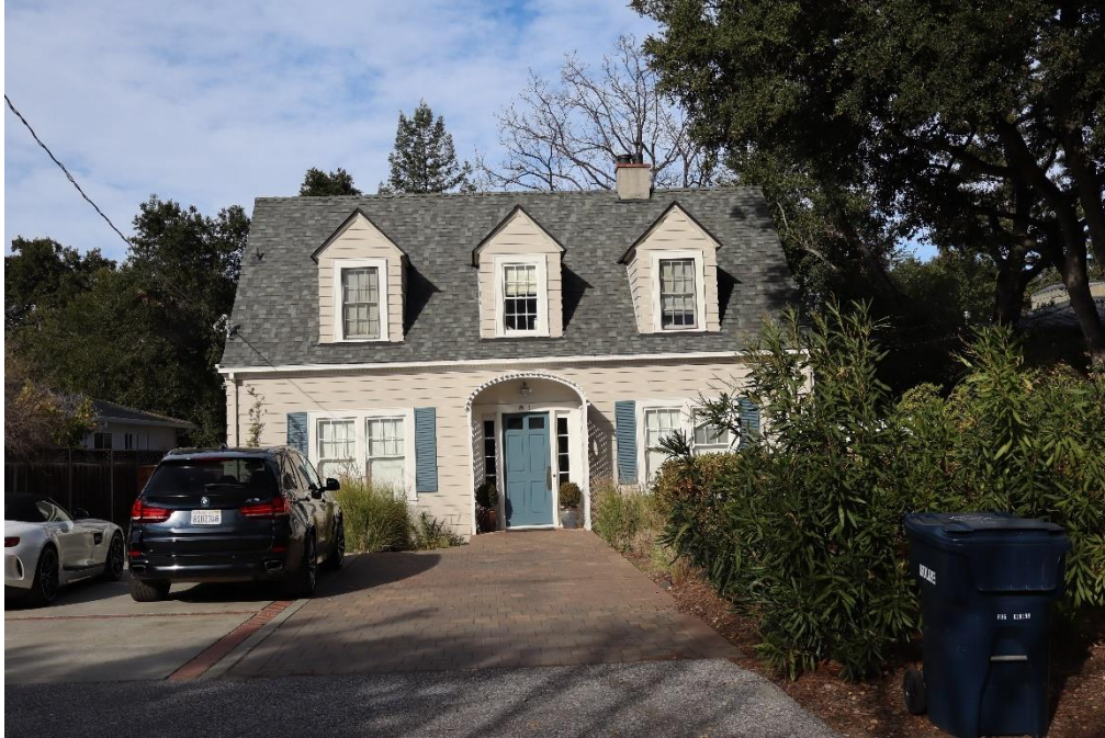
Figure 17. South elevation, facing north.
