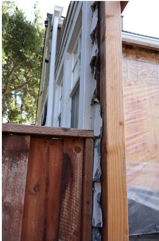
Figure 9. Photograph showing a portion of an addition that was retained as part of a current project.
