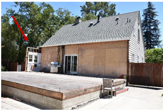
Figure 5. North façade, view southeast. Red arrow indicates east wall of partially removed shed addition
