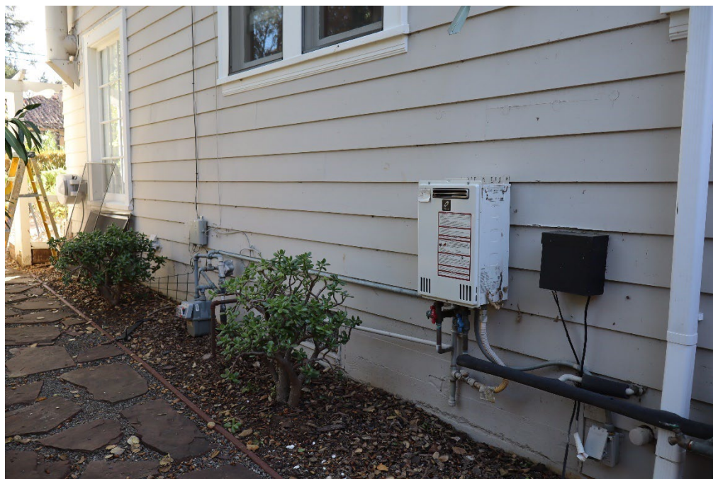
Figure 11. Photograph showing the board-formed concrete foundation is exposed along this elevation.
