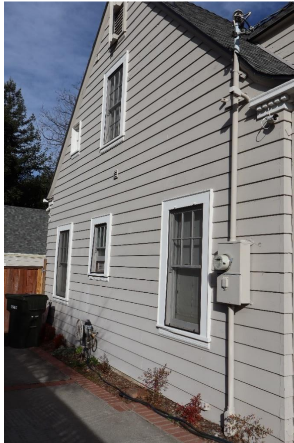
Figure 21. West elevation, facing north.
