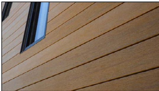
COMPOSITE SIDING (HARDIE PANEL)
